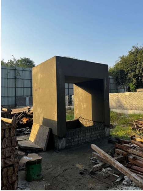
Cutout provided for basement ventilation.
